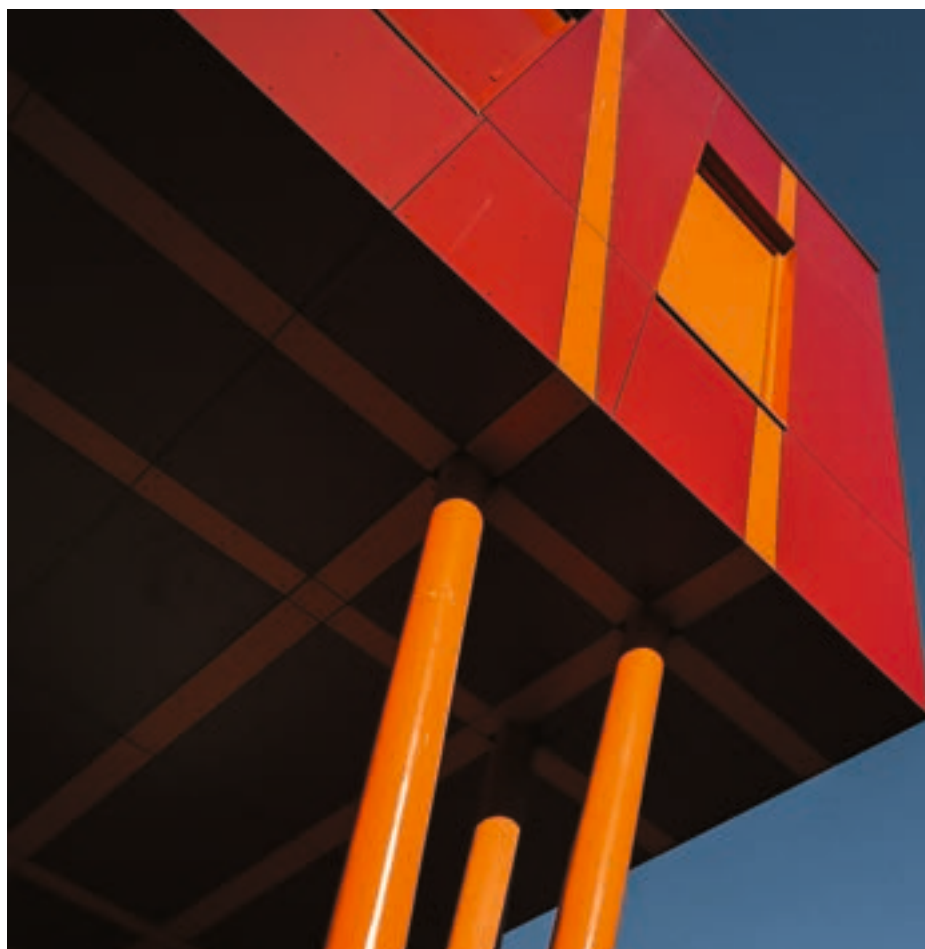
Station de transfert de Joinville
